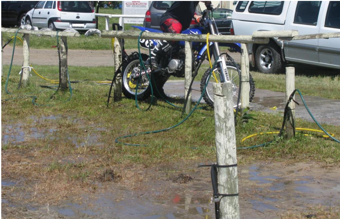
Above: Wash Area without proper drainage. Potential pollution risk especially if located in the vicinity of fresh water sources or in areas with a high water table.
