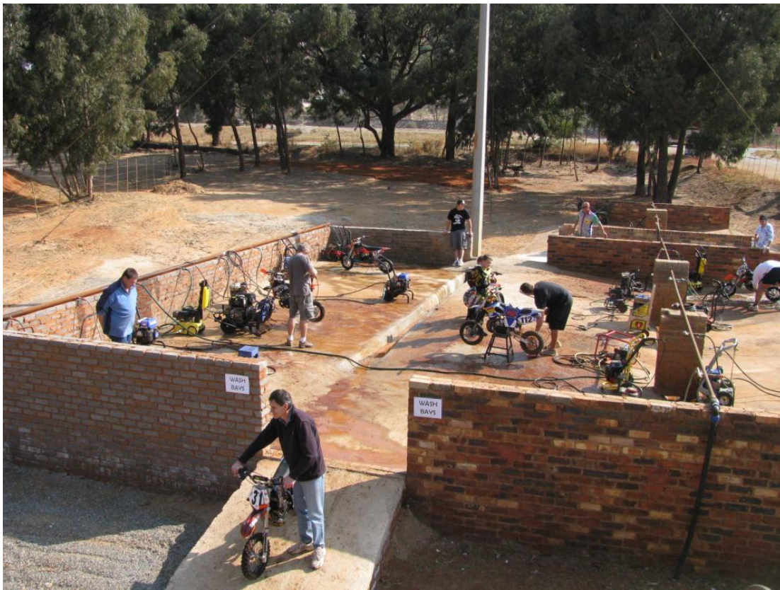
Above: Well designed Wash Bay with concrete floor and controlled waste water disposal system.
