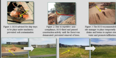
Figure 4: Excessive soil erosion due to construction activities, ECO ensured that grass was rehabilitated and irrigated
