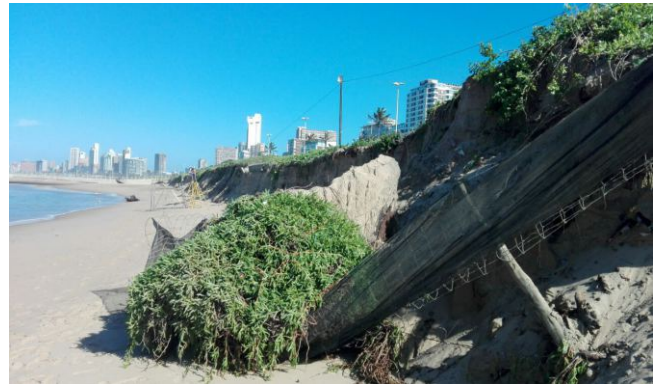
Loss of foredune and coastal access boardwalk at Suncoast Beach, Durban.
