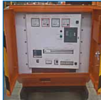
Figure 6, 315kVA dual ratio, 550/400V with MICOM P115 relay
