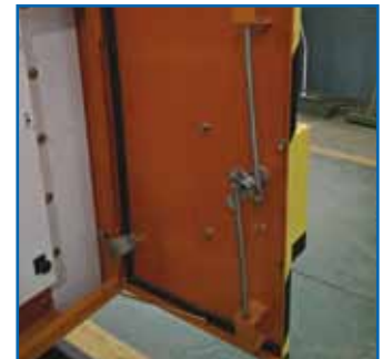
Figure 7, strengthened doors with 8mm rods & barker nelson handles
