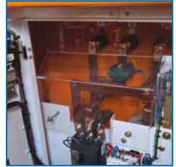
Figure 5, shrouded busbars for zero touch potential
