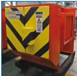
Figure 8, typical LV panel with IP 54 rating
